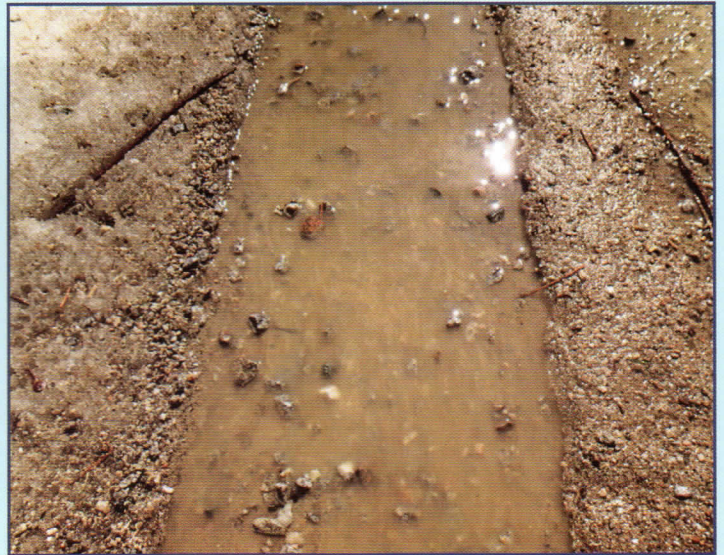
Photo 2: Runoff water from eroded rural roads contains visible sediment and unseen nutrients that can degrade nearby surface waters.
