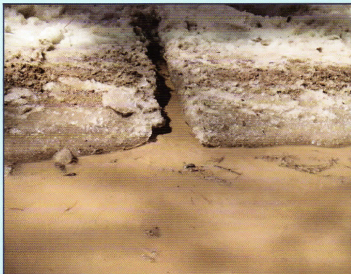
Photo 3: Manually creating narrow splits in ice dams along rural roadways can direct runoff water off of the road, helping to prevent catastrophic roadway washouts.
